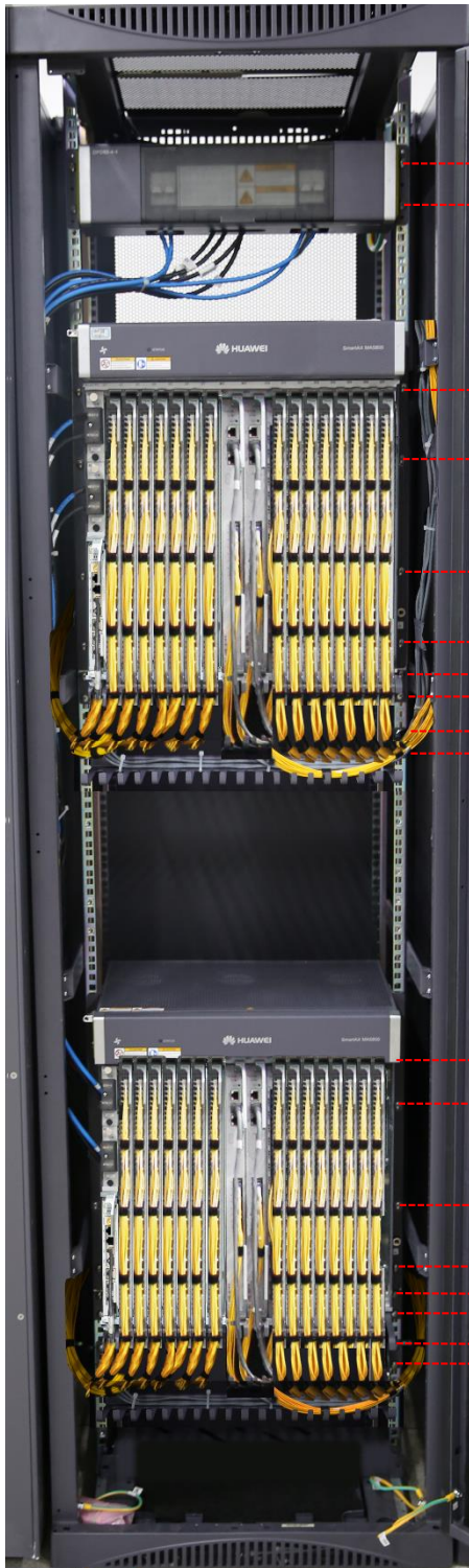
Cabinet configured with 2 MA5800-X15 subracks
