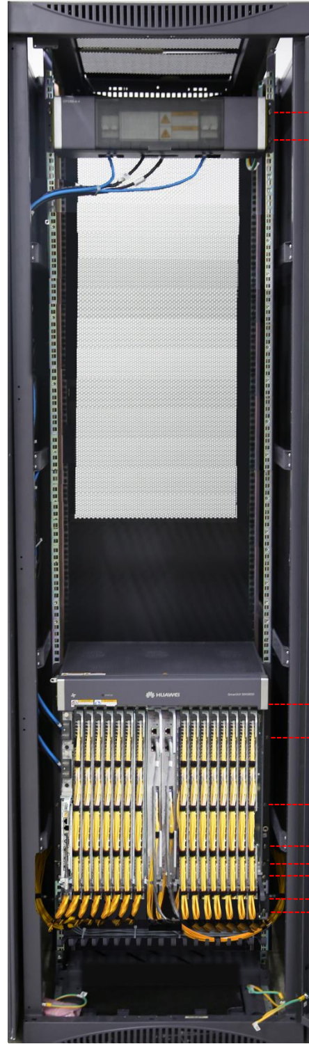
Cabinet configured with a MA5800-X15 subrack
