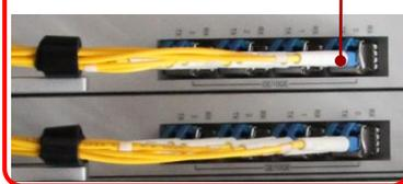
**Mode 2 Routing upstream and downstream optical fibers separately**
